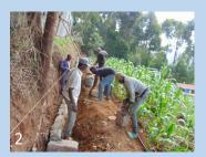
There are two different crews working on this project. One crew is involved in clearing all the trees and bushes in the path of the new fence and constructing the fence. The second crew is composed of masons, who are building an eight-foot-tall wall built with quarry stones around and behind the girls' dormitories.
